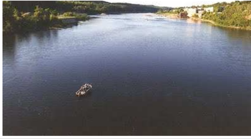
Kennebec River at Augusta, Maine, July 2000, one year after removal of the Edwards Dam. The dam was located in the upper center of the photo.
